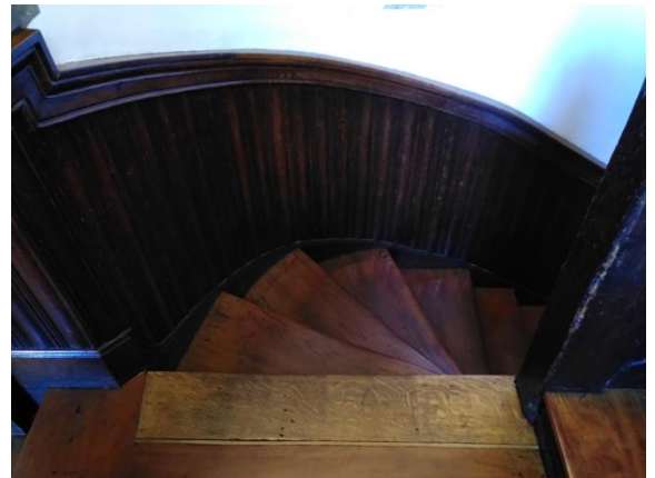
The second flight of stairs curves to the right as you exit the landing area before straightening back up. There is no handrail at this point.
