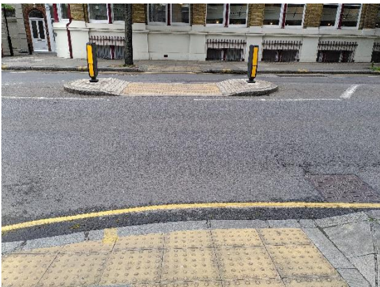
Clerkenwell Road has a pedestrian crossing with dropped kerbs and a refuge island.
