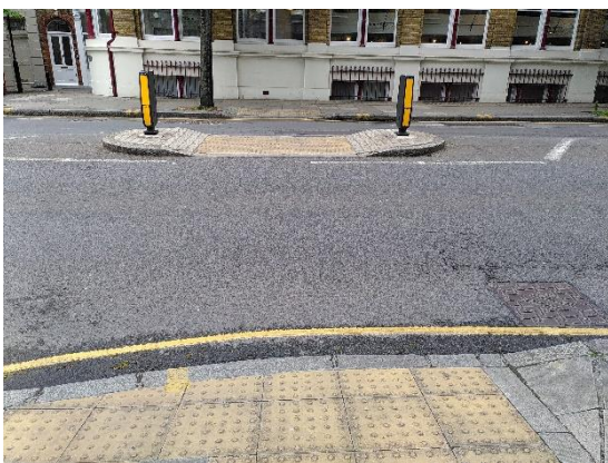
Clerkenwell Road has a pedestrian crossing with dropped kerbs and a refuge island.
