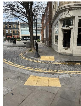
There is a dropped kerb for the crossing over Albemarle Way.
