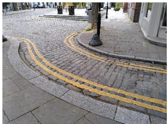
There is no dropped kerb for the crossing over Albemarle Way.
