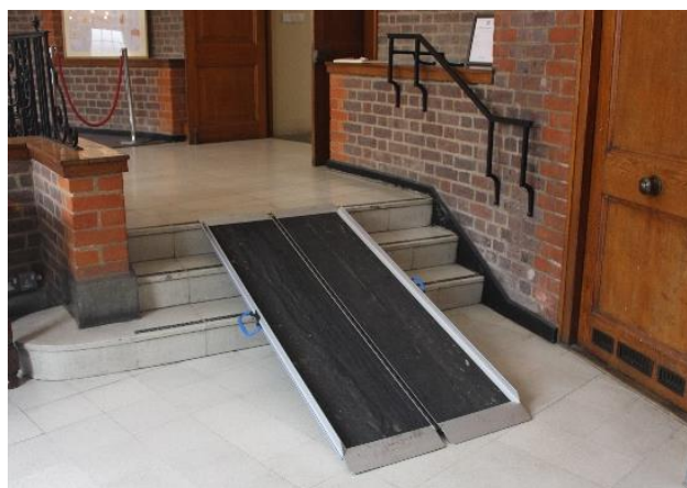
From the Church foyer into the Church, there are 3 steps. A permanent handrail is available on the right as you ascend.
